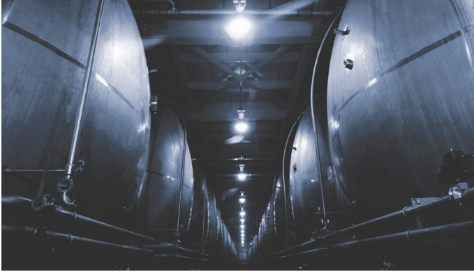
Fill level measurement in tanks
